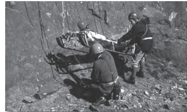
Horizontal lower with control at the top and two barrow boys wearing rope harnesses.
